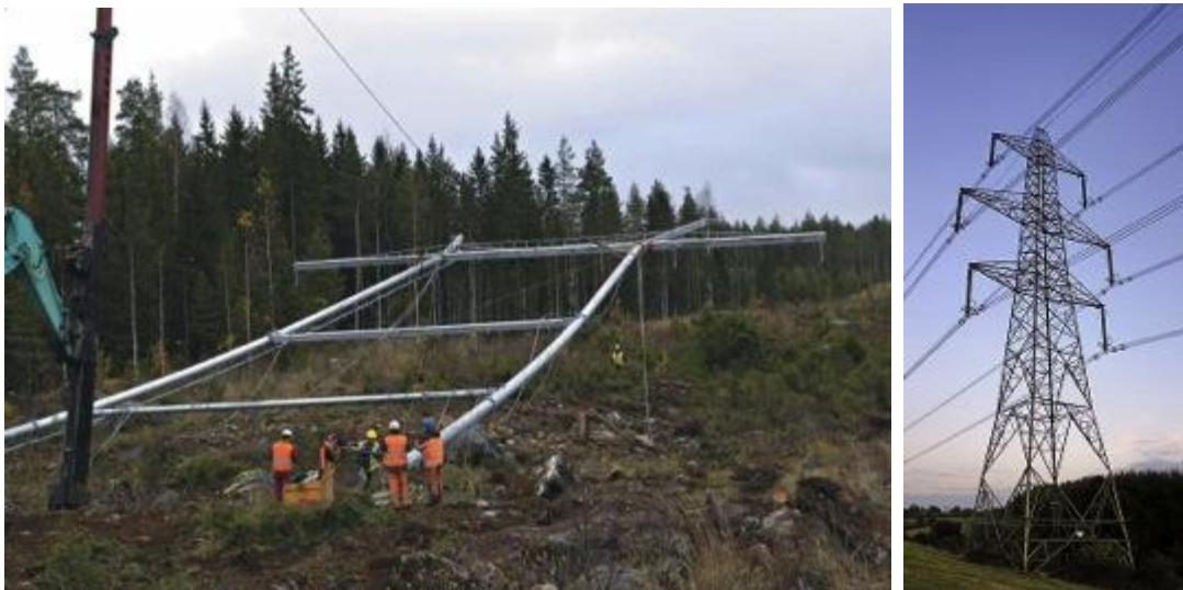
Photo left: construction of overhead powerline on Hill of Aldie, UK © Anne Burgess, Creative Commons, Photo right: two-circuit, single-voltage power transmission line; "bundled" 4-ways©yummifruitbat, Creative Commons.
