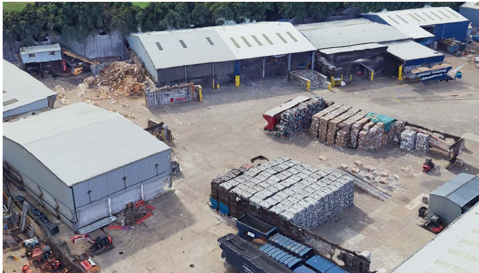
| Veolia's plant in St Albans, UK
